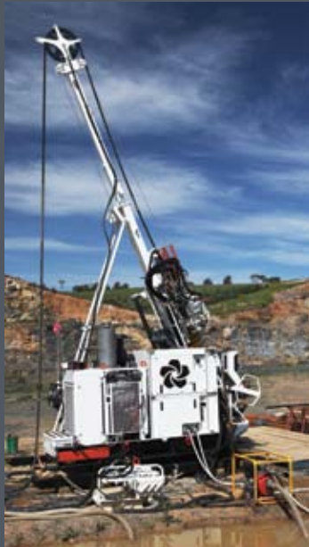
Diamond Coring Rigs
